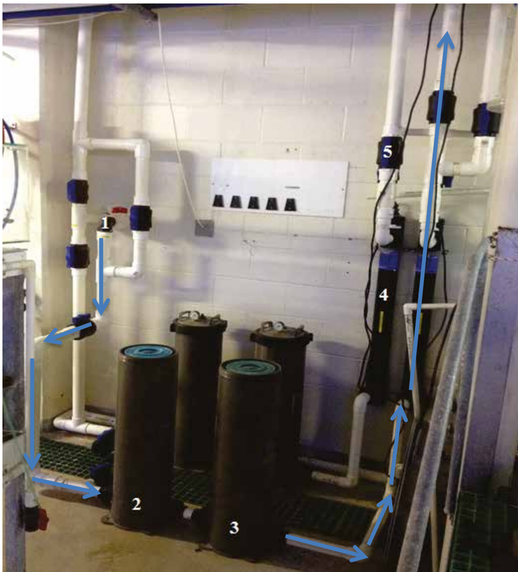
Figure 31. Seawater filtration and sterilisation unit (1) incoming seawater (2) 10 \mu\text{m} filter + housing (3) 5 \mu\text{m} filter and housing (4) UV steriliser (5) outgoing seawater. Blue arrows represent water direction.
