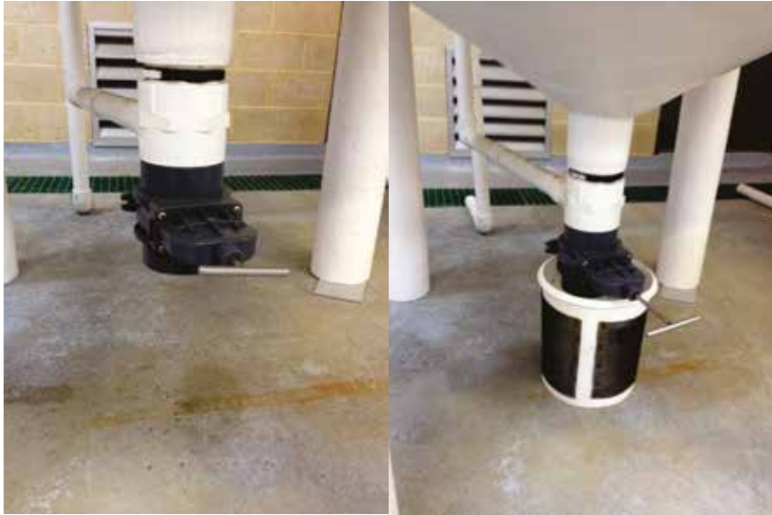
Figure 19. Gate valve with bucket underneath.
